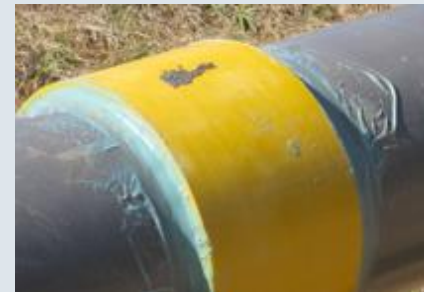
Casing Spacer cut to 5½" in width, installed as casing spacer
