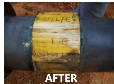
Casing Spacer cut to 5½" in width, installed as casing spacer
