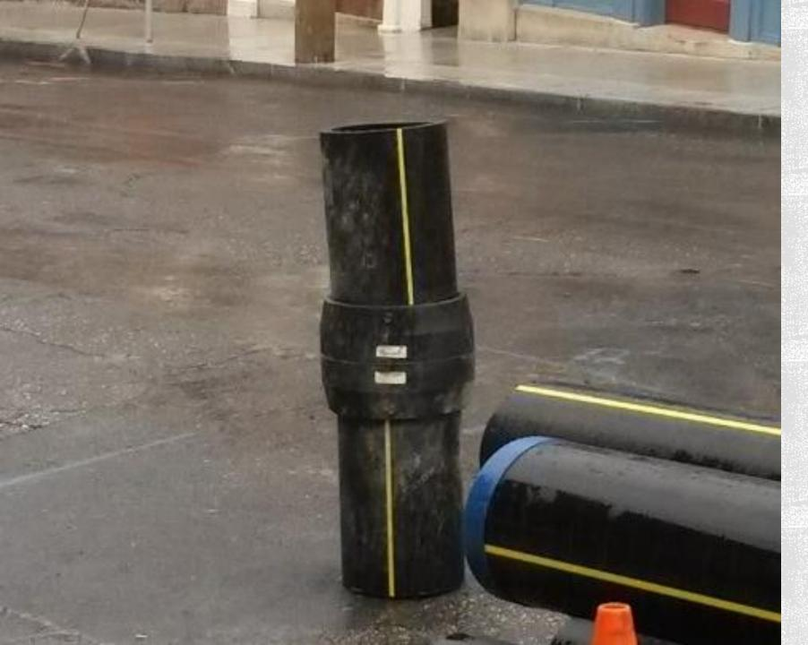
Depth should be marked to insure that pipe/ coupling do not shift during fusion.
